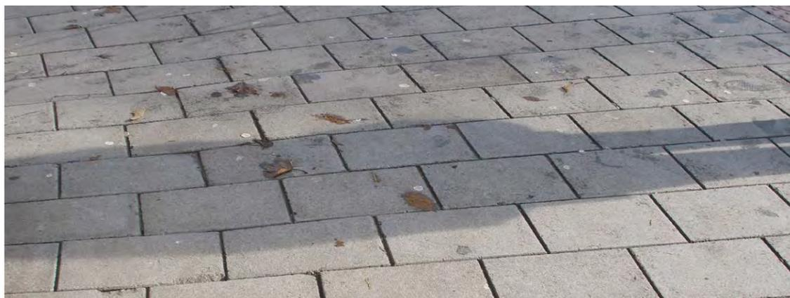
Figure 199: Concrete paving slabs laid in a radial pattern
