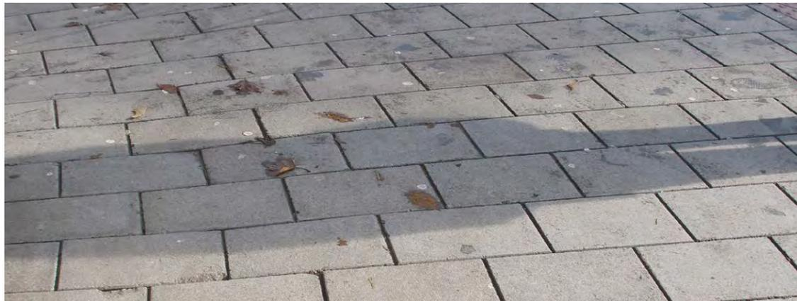
Figure 199: Concrete paving slabs laid in a radial pattern
