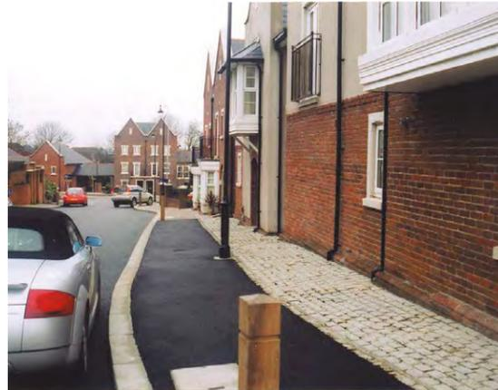
Figure 204: Concrete blocks used on private strip
