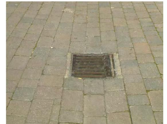
Figure 207: Blockwork drainage channel with grating
