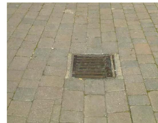
Figure 207: Blockwork drainage channel with grating
