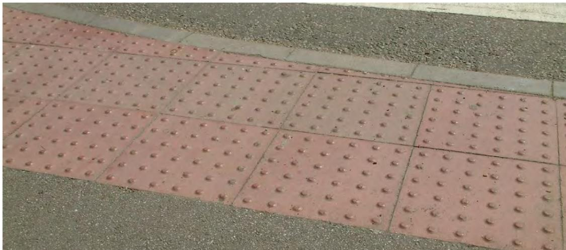
Figure 205: Tactile paving
