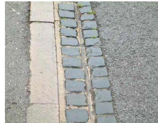
Figure 206: Granite setts used as drainage channel
