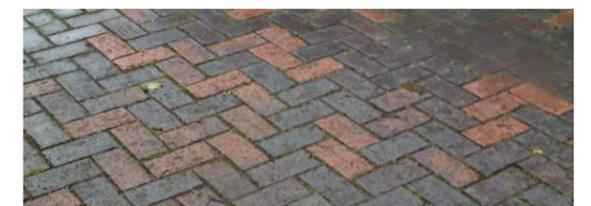
Figure 198: Clay block paving
