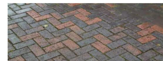
Figure 198: Clay block paving
