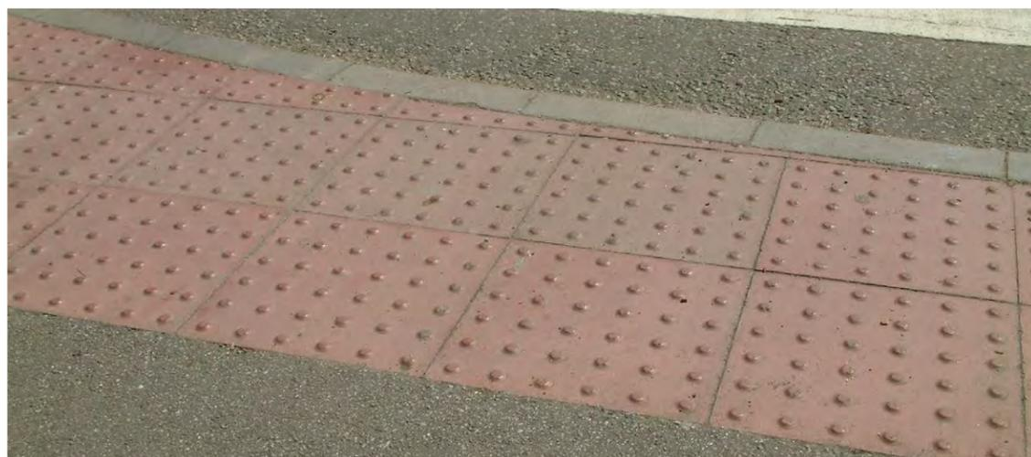
Figure 205: Tactile paving
