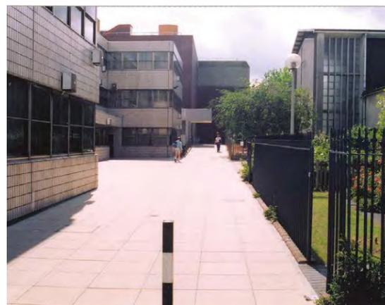
Figure 201: Textured concrete slabs
